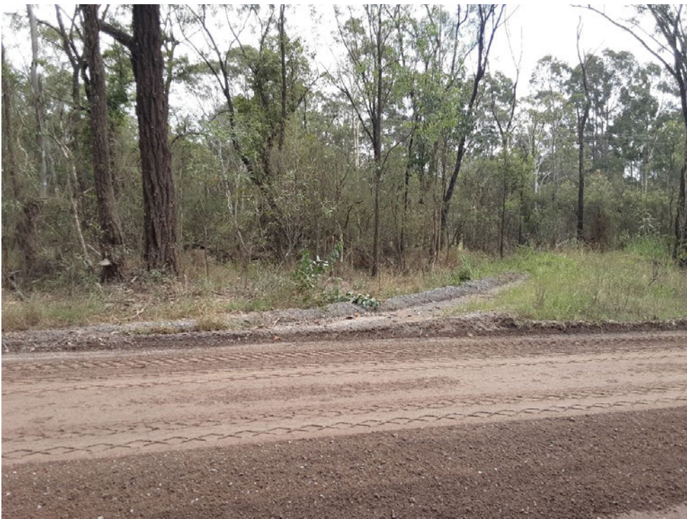
Photo 19 Disturbance associated with road grading and construction; photo taken facing east
