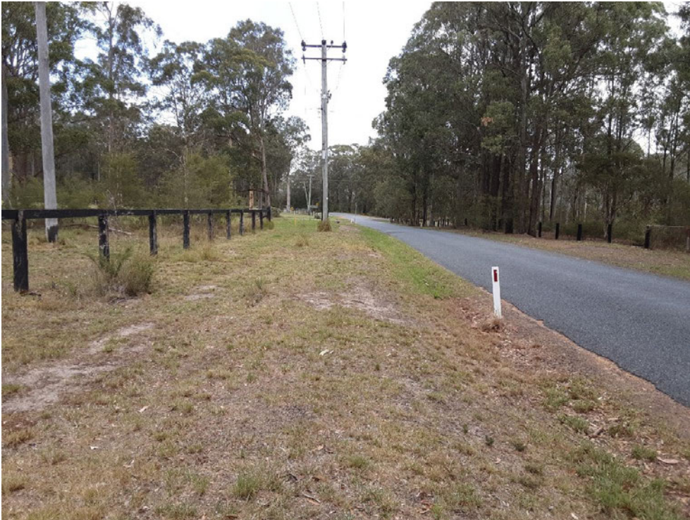
Photo 18 Disturbance associated with electricity installation and fence line; photo taken facing north
